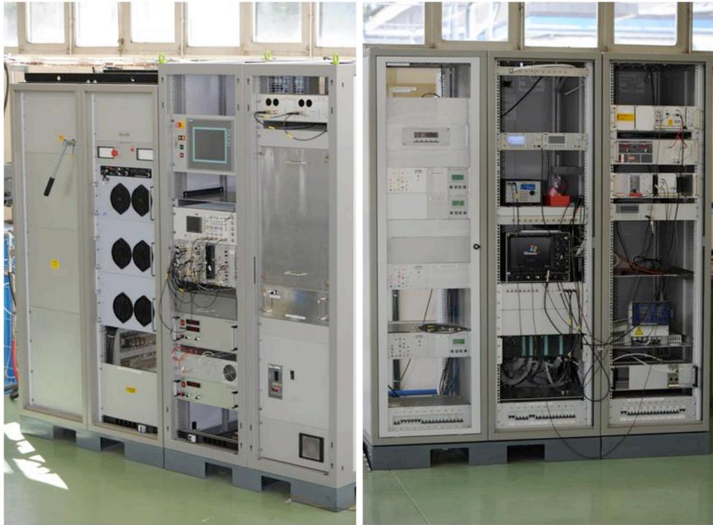
**Figure 35:** Left: High voltage and 2MHz RF generator. Right: Vacuum and controls racks.
