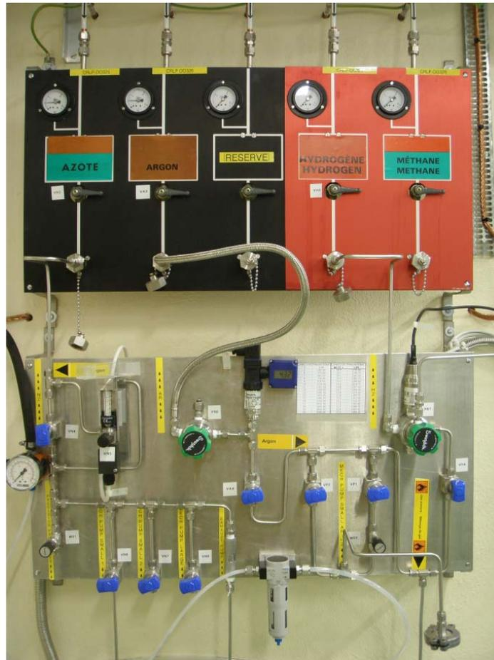
**Figure 29:** Gas distribution system. Top: Patch panel. Bottom: Low pressure gas distribution.
