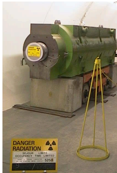
Figure 7: TIDVG internal beam dump
