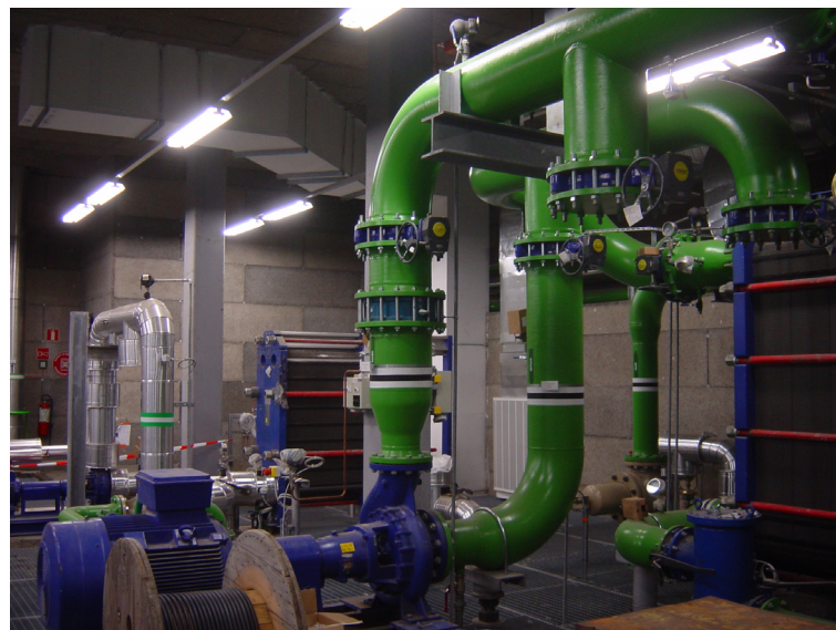
A view of the ATLAS service cavern.
