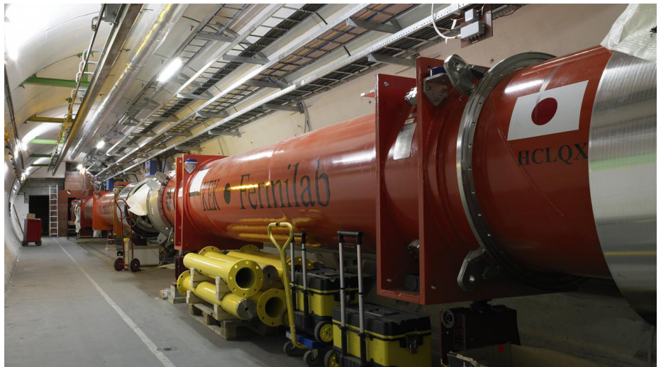
A set of Inner Triplets currently in use in the LHC tunnel.
